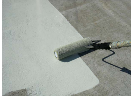
Example: Roller applying 224HS Basecoat
