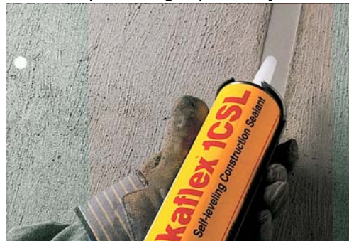
Example: Filling expansion joints
