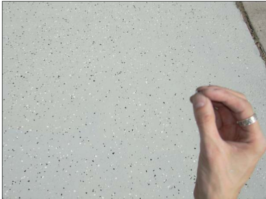
Example: Use a small pinch of color chips
