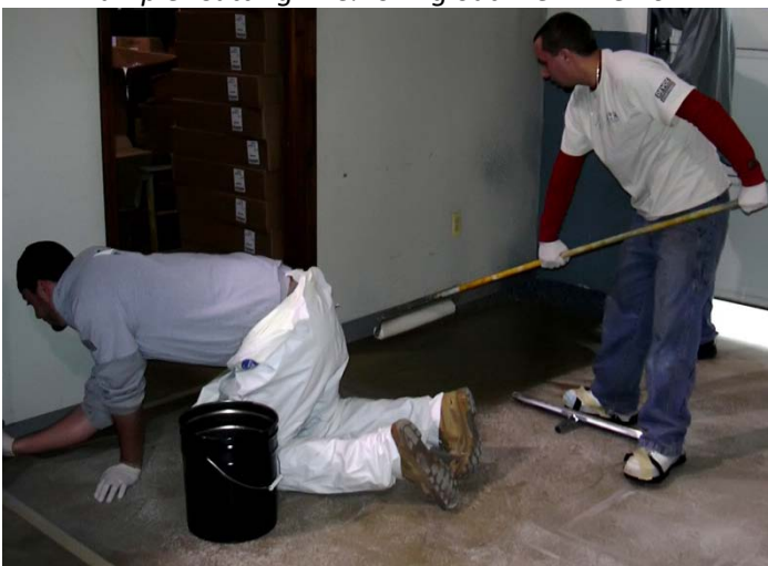
Example: Cutting-in & rolling out PrePrime 167
