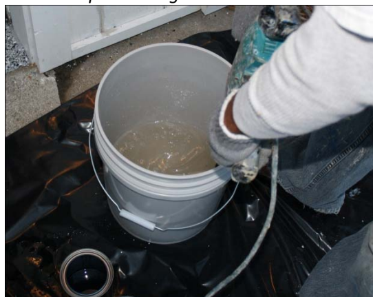
Example: Mixing HPU 747 clearcoat
