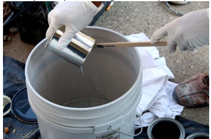
Example: Mix part A & B together in a separate pail
