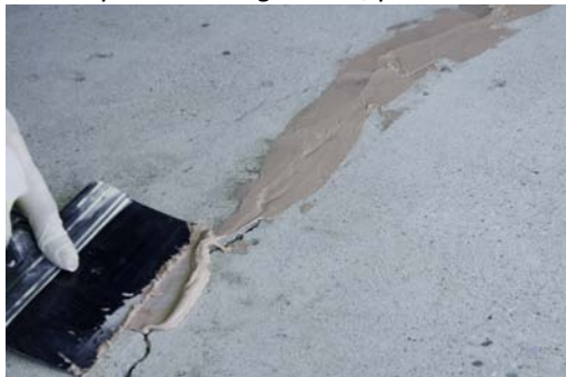
Example: Patching cracks, pits & divots
