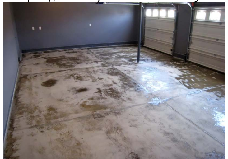
Example: Applied and dry PrePrime 167 Penetrating Sealer
