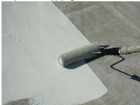
Example: Roller applying Norklad WB Basecoat
