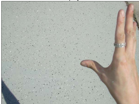
Example: Release and let chips float down onto the epoxy
